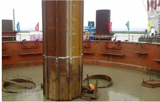
Figure 1. Dredging for piling in Padma rivers for Padma bridge [8]
