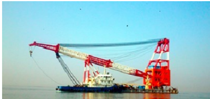
Figure 2. Cutter suction dredger used in dredging for Padma Bridge [8]
